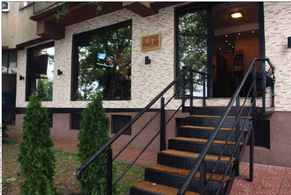
Entrance to C7 Restaurant
