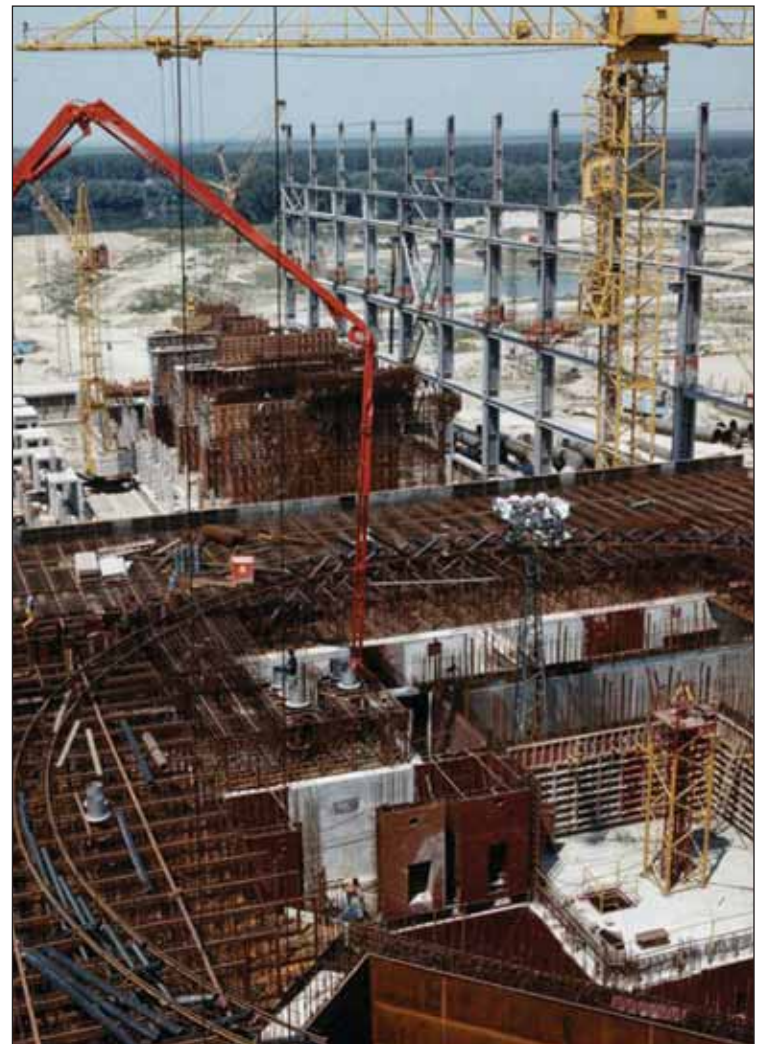
The Belene nuclear power plant
