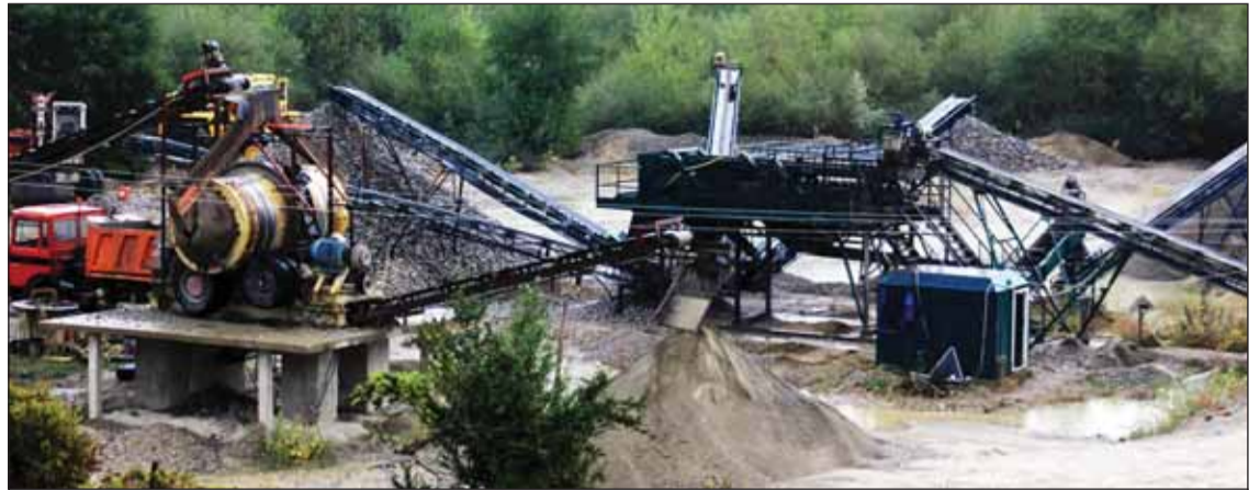
Diggers at work illegally exploiting the Drini river.
