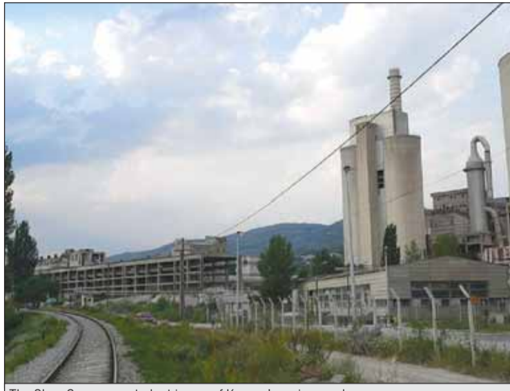
The SharrCem cement plant is one of Kosovo's major employers
